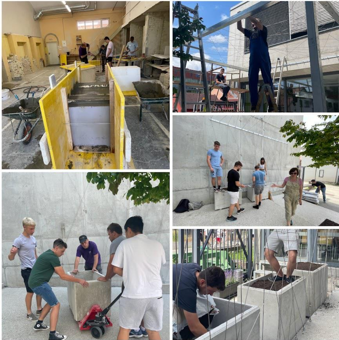
Figure 9 Work in progress – realization of the project (own source: TPN)
